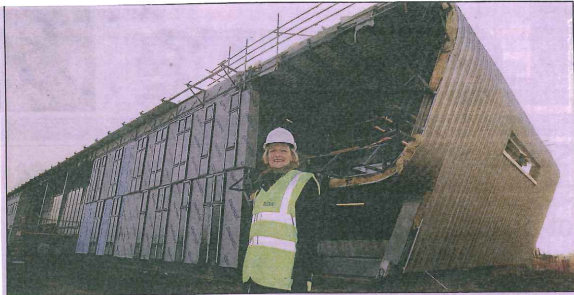
■ Forging ahead – headteacher Jean Alder on the construction site
